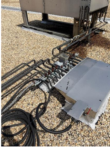
Figure 9: Existing Pipe and Conduit Roof Portal
